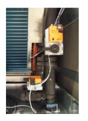
2-way motorized valve with 0÷10 VDC control actuator and emergency manual control for the third way (by-pass) of the hydraulic circuit.
