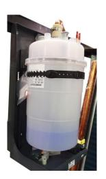
Modulating steam humidifier with immersed electrodes fitted with safety and running accessories. The optional includes the combined temperature / humidity sensor on unit air intake. The optional is not available for size E1, E2.
