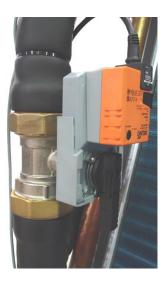
The water flow control in the finned coil is acieved through a **2-way modulating ball valve with equal percentage flow control** ensured by the integrated characterizing disc.
